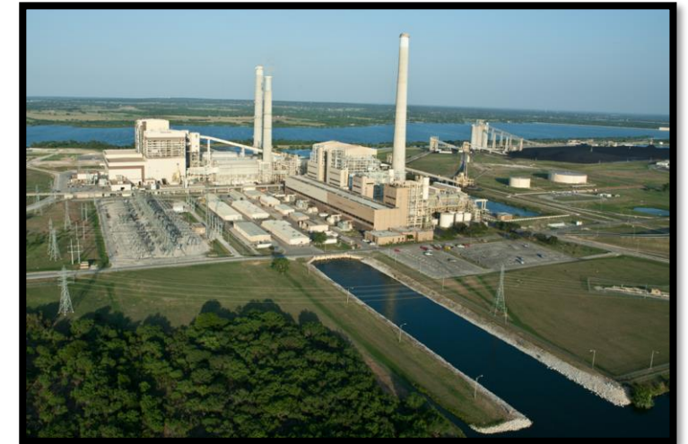
Spruce 1 & 2 Coal Plant Built in 1992 & 2010 1345 MW
