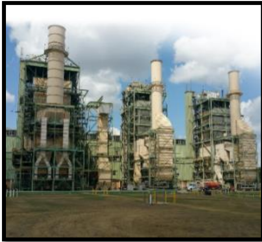
Braunig 1, 2 & 3 Gas Plant Built in 1966, 1968, 1970 859 MW
